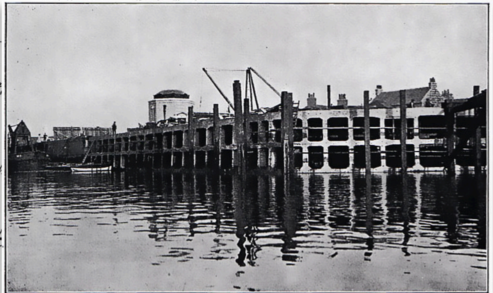
ABERDEEN HARBOUR EXTENSIONS: NEW WHARVES Engineer, Mr Gordon Nicol, M.Inst.C.E.
